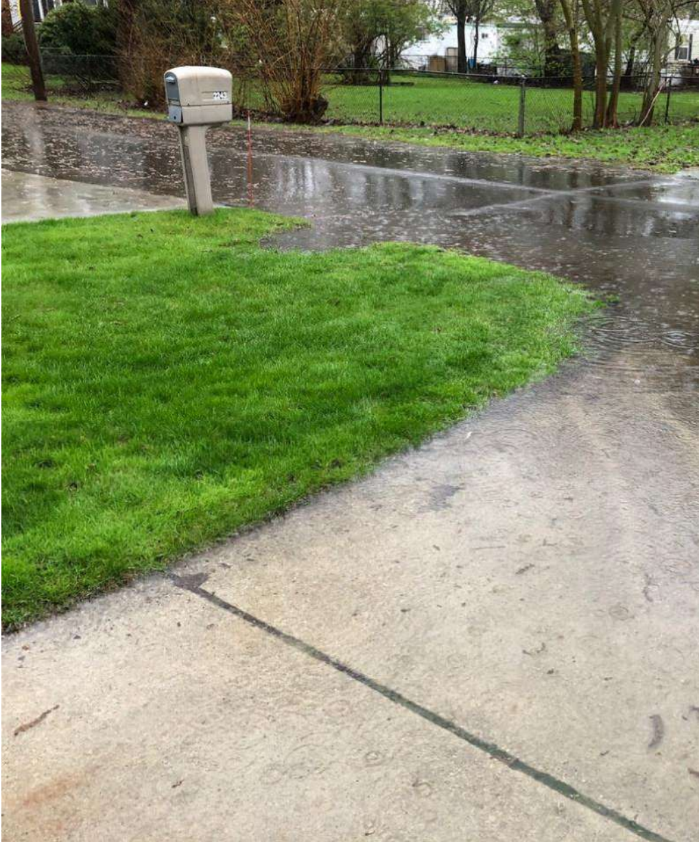
Photo from homeowner at 2229 Willow Beach St from May, 2019 of the flooded driveway and street.
