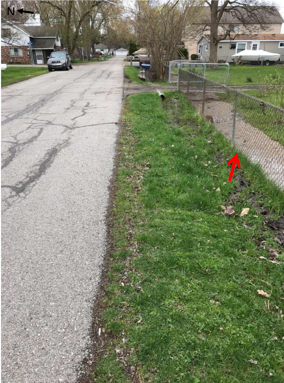
Image taken by HRC staff on May 3, 2019 of the heaved culvert at 3201 Kenrick and the location where the homeowner of 3201 Kenrick placed a sand berm to prevent roadway runoff from draining to their property.
