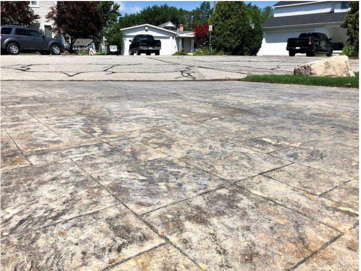
Elevation comparison of driveway compared to the road from July 30, 2019, taken by HRC staff.
