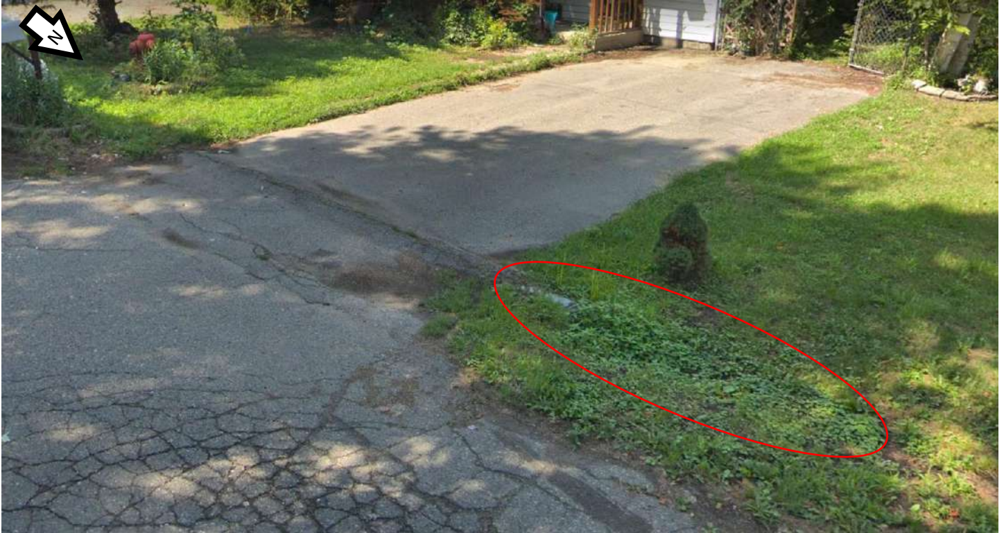
Buried culvert and ditches.
