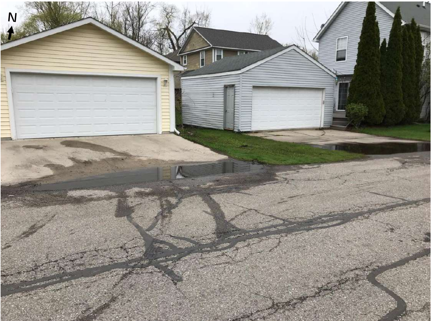
Image taken by HRC staff on May 3, 2019 of standing water at driveways of 2141 Willow Beach Street and 2140 Brock Street.
