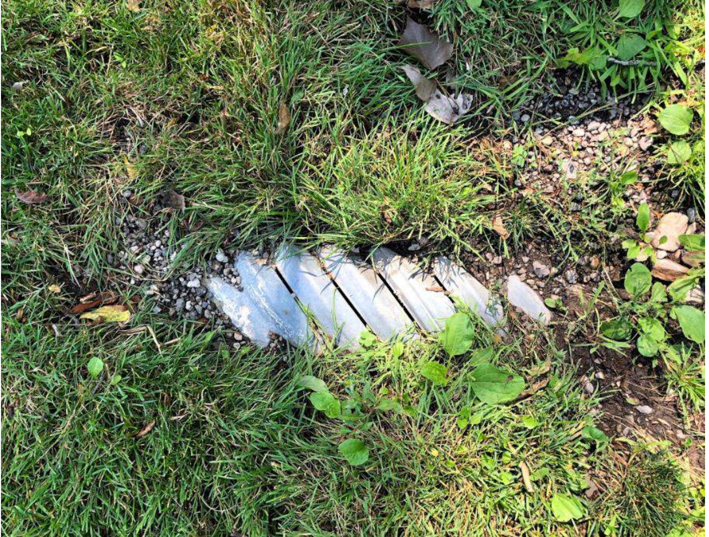
Photo taken by HRC staff the exposed drain and slit created to allow flow into the pipe from July 30, 2019. Location where field catch basin is recommended to be installed.
