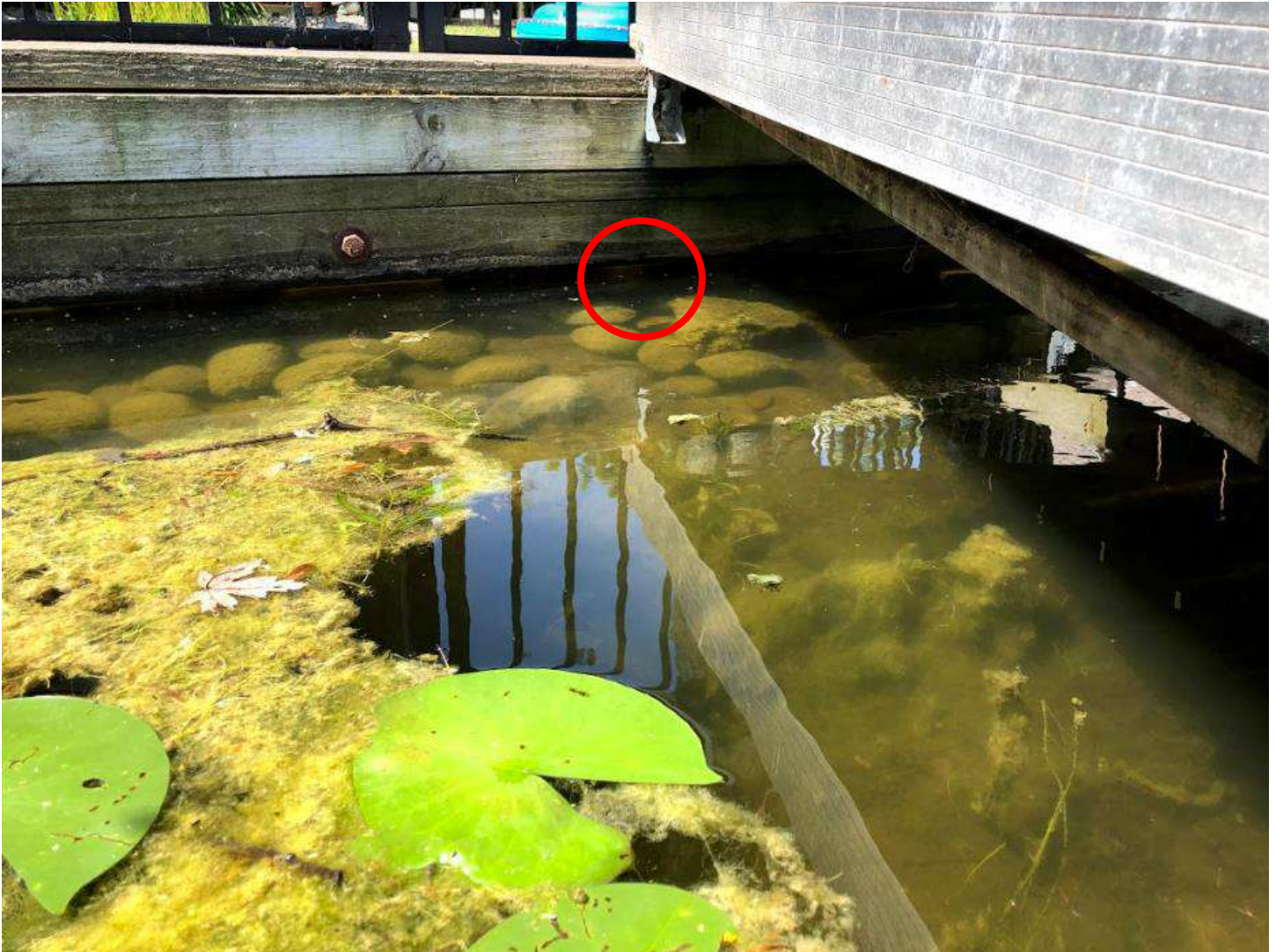
Photo taken by HRC staff of culvert outlet through the seawall into Sylvan Lake.
